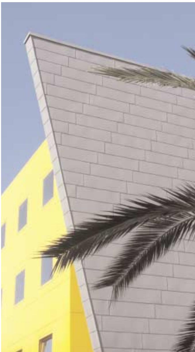
The Flat Lock system can be installed on flat and gently curved façades.
