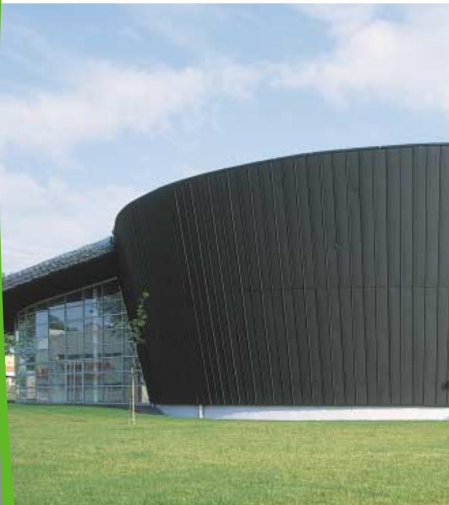
From its original function, standing seam has flowed down to clad the façade, wrapping the building in a continuous unifying envelope. The use of standing seam gives continuous joints from the roof to the façade while guaranteeing maximum watertightness. Of course, this technique can also be used for the facade only...
